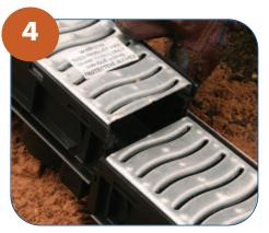
Join two lengths of channel by interlocking them at each end.
