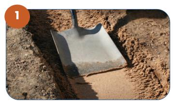
✓ Dig trench for FloDrain, allowing for 50mm deep compacted sand base and wide enough for a minimum of 100mm backfill of concrete on each side.
