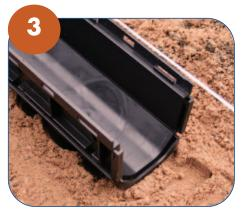
Start installation at lowest point of the run to accommodate any cut lengths which should be installed at the point furthest from the outlet.
