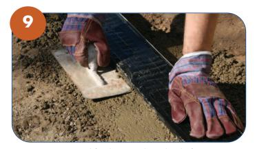
Pour concrete and finish 2mm above level of grate.
