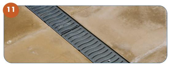
✓ If installing block paving or paving slabs, haunch around channel with concrete to a height which allows the depth of the block or slab to finish 2mm above the level of grate.
