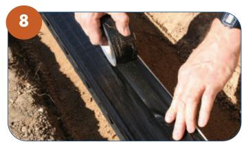
✓ Protect grate with tape before concrete is poured.
