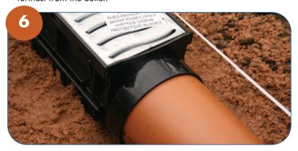
Connect the lowest end of FloDrain to 110mm PVC-U BS EN1401 drainage pipe using either an end outlet or the preformed channel bottom outlet to allow water to drain away.
